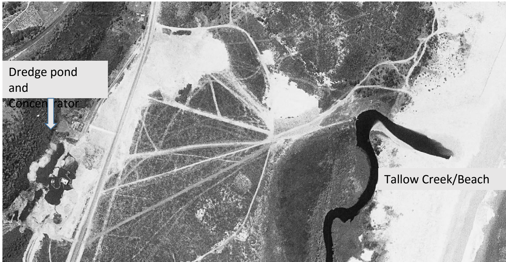
Mining at future Red Devil's sports ground and high school – 1966. (Photo – NSW Govt)
