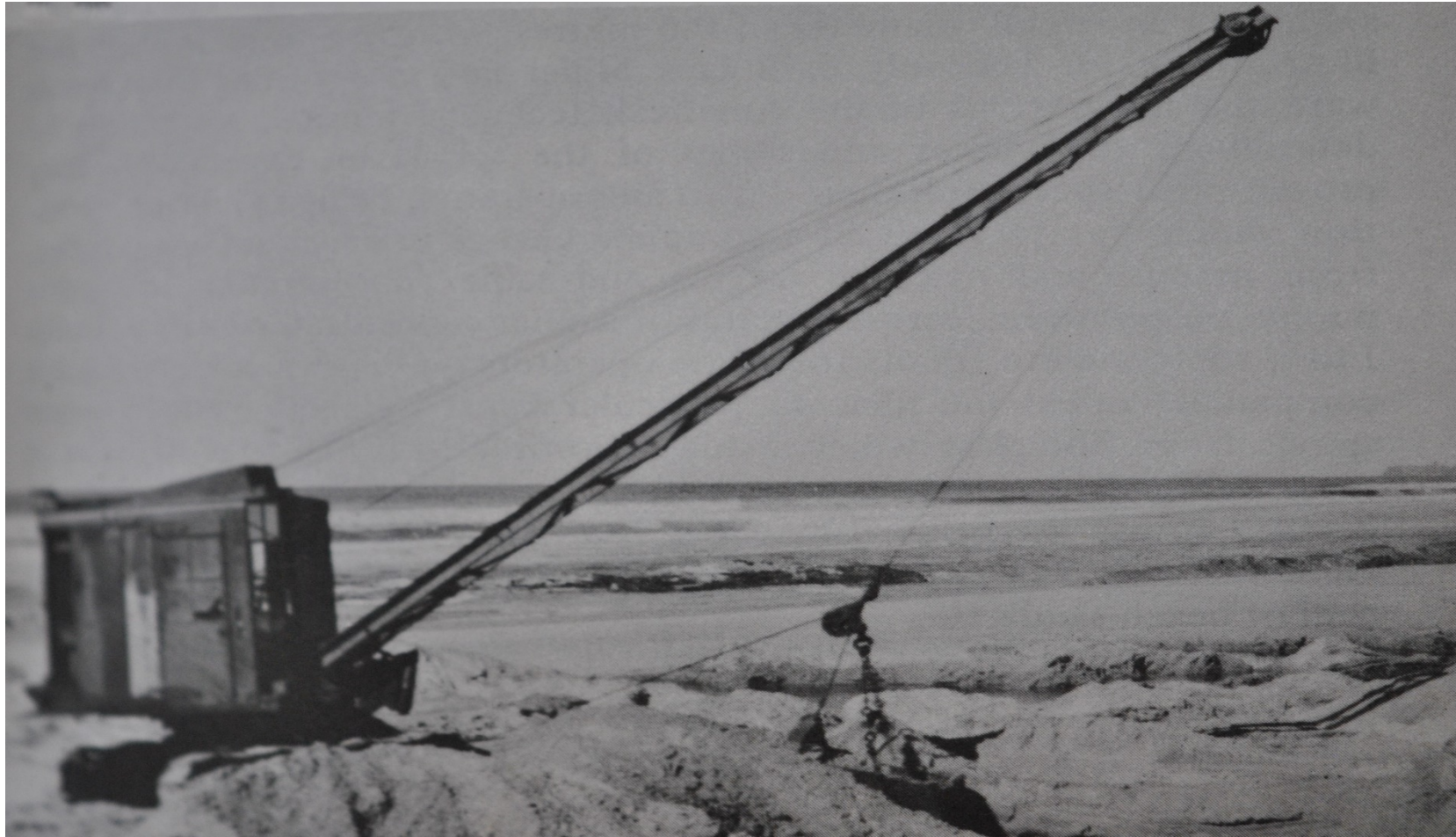
Primitive dragline mining sand - Seven Mile Beach mid 1940's. (Photo - Morley)
